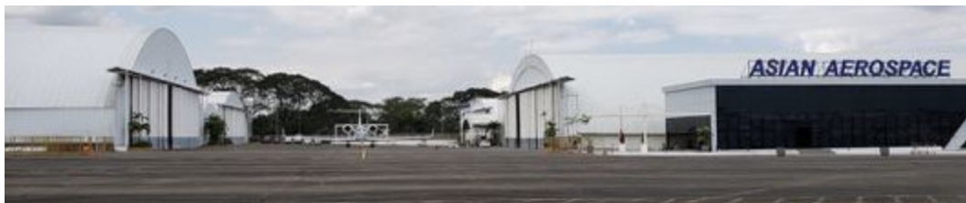
Fig. 11: Ground view of Asian Aerospace hangars.
